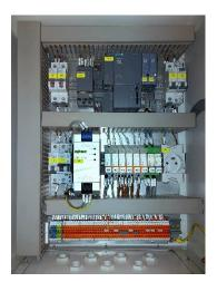
Thanks to such a combination, the user receives data packets in the network protocol containing data on the level of the tested material and/or data enabling the creation of visualization on the user's existing PLC system. Data can be sent in any network protocol (Ethernet, Profibus, Profinet). Also as an option, the user can set the desired activation levels of the relay outputs (2 relay outputs warning and exceeding zone).
